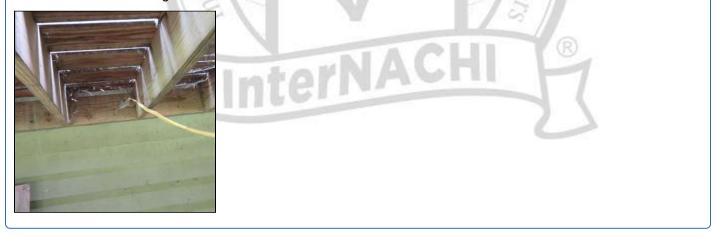
**2.3** (3) Did not observe any concrete posts or pads under support columns for original deck. Recommend further inspection and if posts are not on concrete I recommend concrete pads be installed under all posts to extend useful life of posts.
