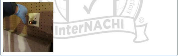
**6.4** (3) Exterior receptacle by door to deck GFCI protected and tripped when tested. However, unable to locate GFCI the receptacle is protected by. Recommend GFCI receptacle be located so it can be reset.
