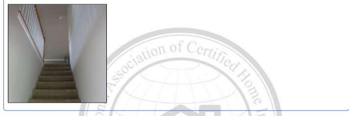
**9.3** (3) Recommend a handrail system which complies with current safety standards be installed for the stairs to the basement.
