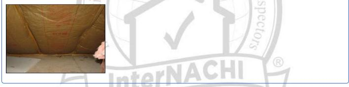
**8.0** (3) Two layers of fiberglass batt insulation in attic, for total of approximately 12" to 14". The R-value of fiberglass insulation is approximately 3.1 to 3.4 per inch.
