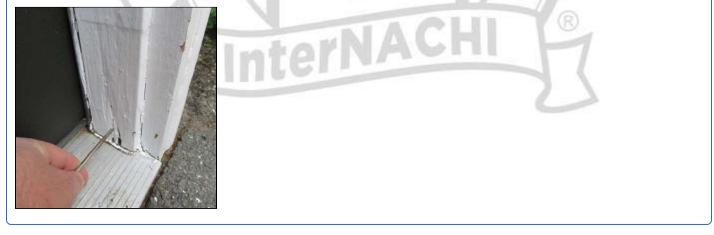
**10.4** (2) Gap between trim on left side of entrance door to garage and missing paint on section of the trim for door. Recommend gap be sealed and any bare wood be primed and painted to prevent moisture intrusion.
