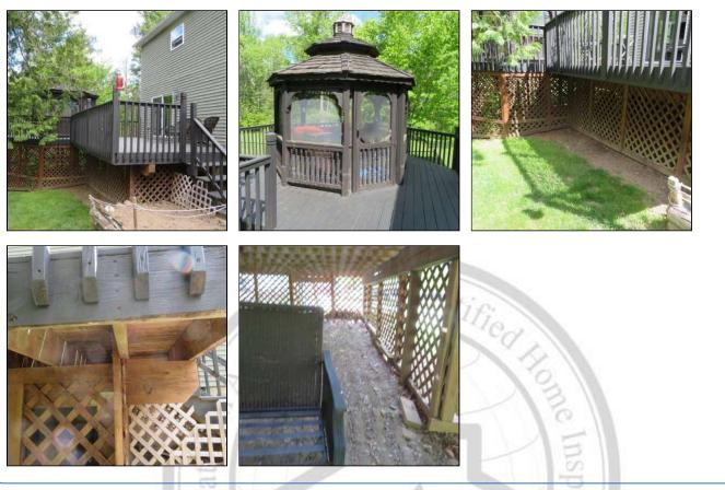
**2.3** (2) Did not observe any bolts fastening ledger board for deck. Recommend lag bolts or other fasteners be installed to secure the ledger board to the house.
