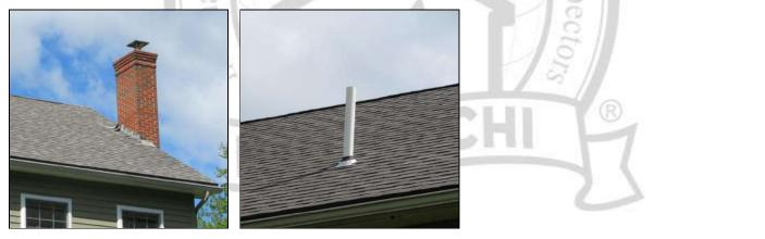
**1.3** (2) I recommend a cap be installed for the entire chimney top, to keep rain, snow, animals and debris from getting into the chimney and possibly damaging the liner or chimney.
