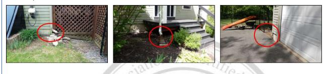
**1.1** (3) Recommend client consider installation of additional gutters on front side of garage, with proper downspouts and extensions, to shed water away from property to avoid erosion and/or water intrusion.
