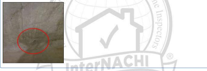
**3.1** Minor cracking in basement wall(s), but no evidence of any structural issues. Cracks of this type are common Recommend cracks be monitored and if any 1/4" or larger that they be sealed.
