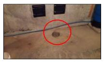
**3.3** (2) Minor cracking in basement floor, but no evidence of any structural issues. Cracks of this type are common. Recommend cracks be monitored and if any 1/4" or larger that they be sealed.
