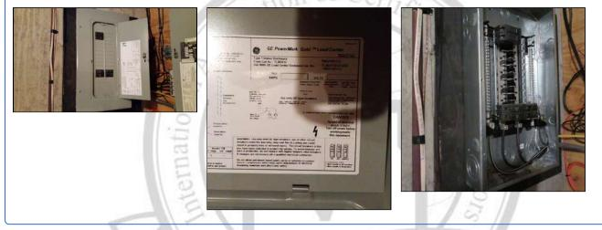
**6.1** (3) Open knockout hole(s) on bottom of main service panel. Recommend proper plug/cover(s) be installed to prevent intrusion of pests and/or moisture.
