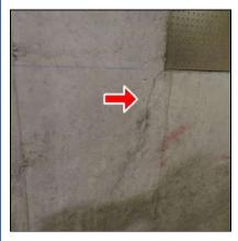
**3.3** (1) Floor drain in basement to right of the boiler. Did not observe where the floor drain pipe terminates. Recommend client(s) run a hose in the drain to determine where it exhausts and if it is functioning. Also recommend a perforated cap be installed on the drain pipe to keep it from getting clogged and to keep animals out of the pipe.
