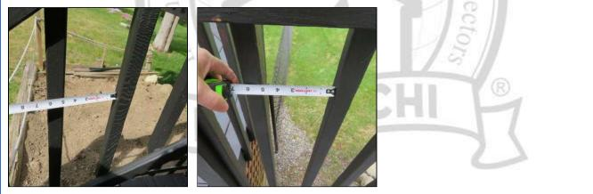
**2.4** (3) Railing systems for steps to deck and sections of railing system for deck are loose in areas. This is common for railing systems as they loosen over the course of time. Recommend the railing system be tightened or repaired as necessary.
