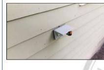
**6.3** (3) Recommend dome covers be installed for all exterior receptacles to protect connection if cord plugged into receptacle.
