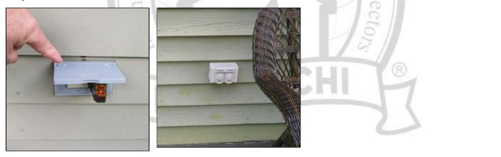
**6.3** (4) Extension cord used to supply power to gazebo. Extension cords are not supposed of be used for permanent wiring. Recommend wiring to gazebo be hard wired and that any receptacles in gazebo be GFCI protected.
