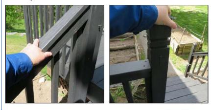
**2.4** (4) Railing system for addition to deck where gazebo is located is approximately 34" tall. Recommend guardrails be repaired to meet the current minimum height requirement of 36".
