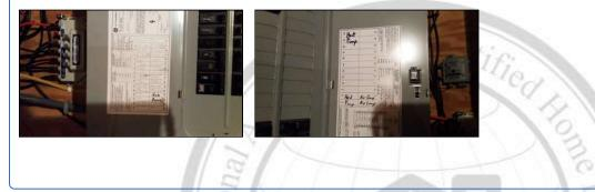
**6.2** (2) Several GFCI circuit breakers. Recommend the GFCI circuit breakers be tested periodically to determine if they are functioning properly. Please refer to Section 6.4(1).
