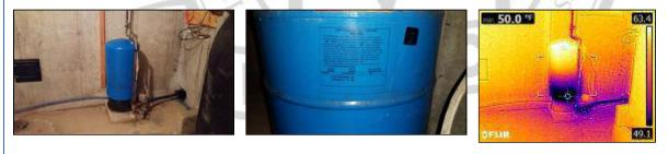
**13.1** (2) Unable to read the water pressure gauge at the base of the air pressure tank in the basement. Recommend the gauge be replaced so the pressure can be determined as part of a routine maintenance schedule or for servicing purposes. The generally acceptable limits for well water pressure at a residence is between 40 PSI and 80 PSI. I tested the water pressure at the exterior spigot. Please refer to Section 2.9.
