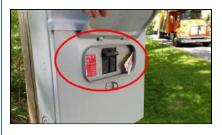
**6.2** (1) Recommend client confirm accuracy of labeling of circuit breakers and that all circuits be labeled. Three Arc Fault Circuit Interrupter (AFCI) circuit breakers in main service panel marked for the bedrooms. Recommend the AFCI circuit breakers be tested periodically to determine if they are functioning properly.
